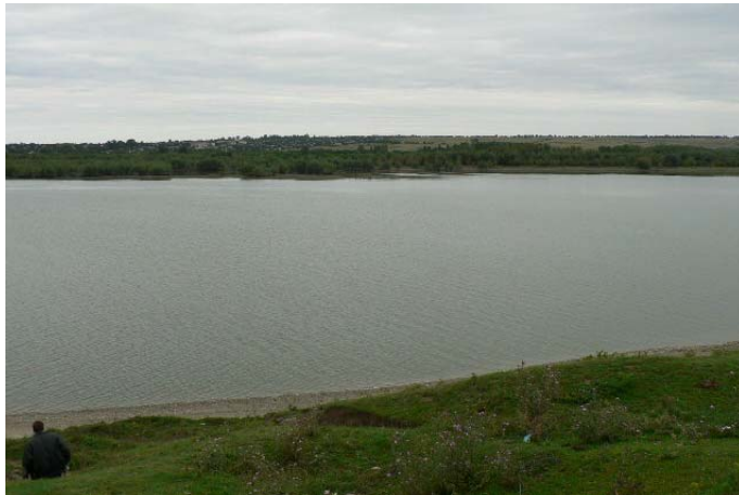
Fig. 2. General view of the Negreni reservoir, Botosani County.
