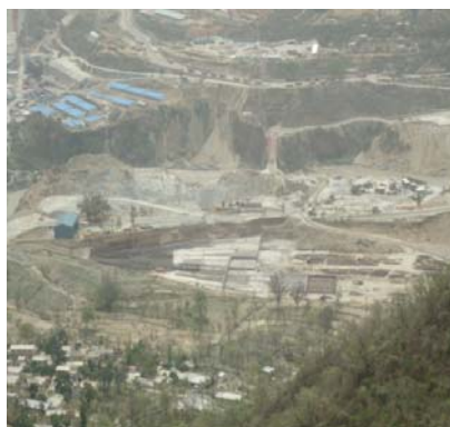
Fig. 3. Dam canal excavation changing existing land pattern
