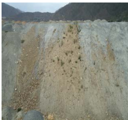
Fig. 4. Dumping of canal excavation material
