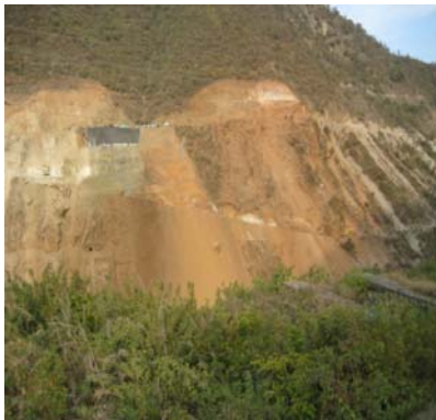
Fig. 7. Forest disturbance in dam road construction
