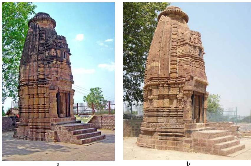
Fig. 1. Sita Devi Temple: a - before conservation; b – after conservation
