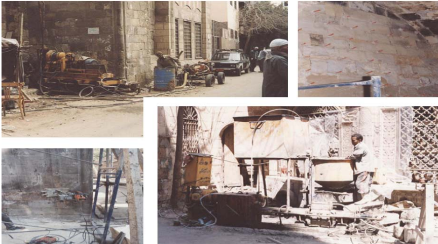
Fig. 5. Gonblat Mosque, Kutab and Sabeel in Cairo. Grouting and injection processes.
