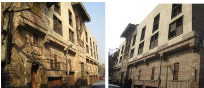
Fig. 9. Rabaa, Kutab and Sabeel Al-Qazzlar after restoration processes
