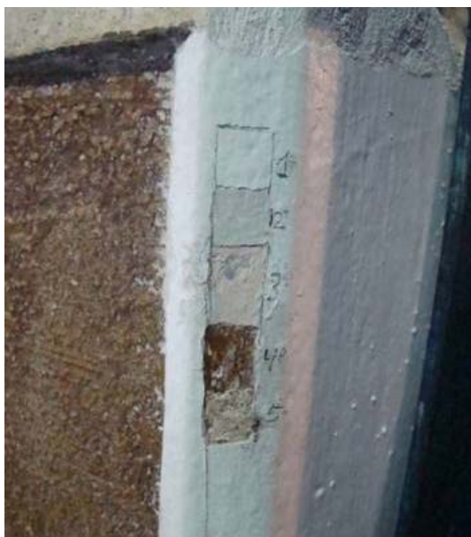
Fig. 3. Stratigraphic windows referring to the five layers found at the historic house under study
