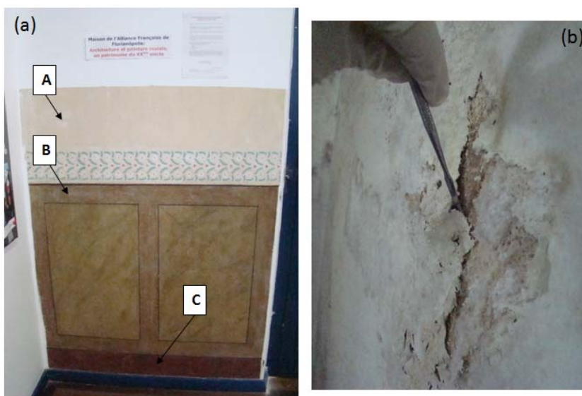
Fig. 2. (a) Mural paintings found at the historic house after pickling of the most recent ink layers; where A is the trace of green painting found in the ornament above, B and C is the ochre and dark brown color respectively (b) traces of soluble salts found during the process.
