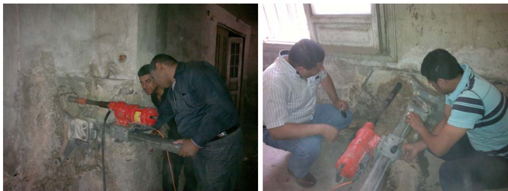
Fig. 4. The Core Samples extraction from the basement of the palace
