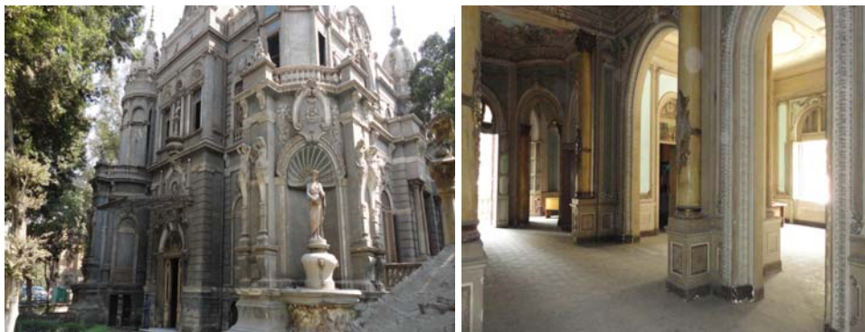
Fig. 1. Sakakini Palace in Cairo, Egypt.
