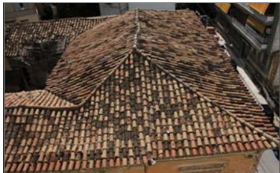
Fig. 5. Roof of Aktaiou building
