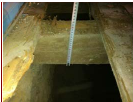
Fig. 4. Floor wooden beams
