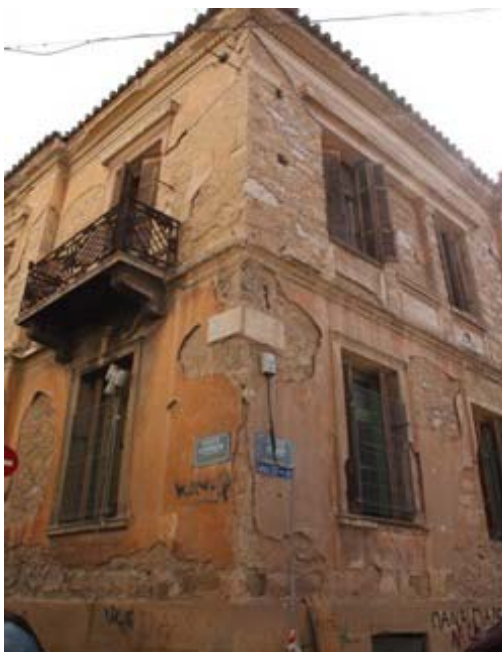
Fig. 2. The Aktaiou building
