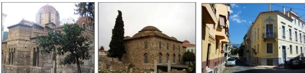
Fig. 1. Typical historic buildings in the Plaka district (Church, Mosque, and traditional houses)
