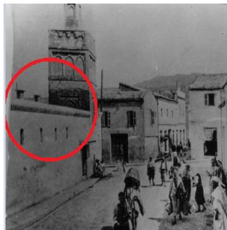
Fig. 6. Change of the Sidi El Benna Mosque roof
