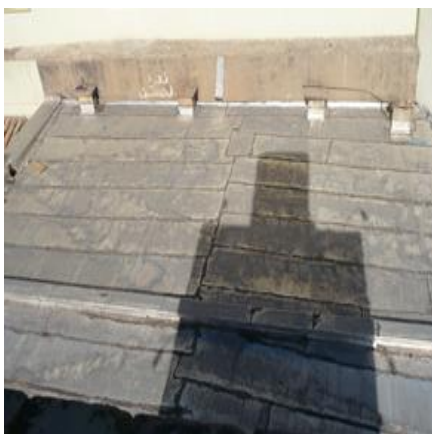
Fig. 9. Aluminum sealing plates on the terrace of the prayer room
