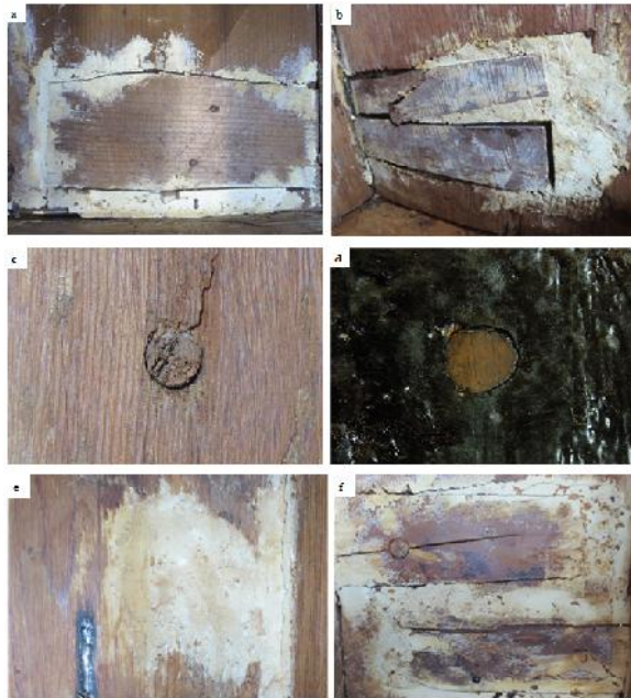
Fig. 8. Methods of repairing and patching wood. a. Patching with another piece of wood secured with dowels and white paste GEM-No 21061. b. Patching with another piece of wood secured with white paste GEM-No 21062. c. Knots holes filled with wooden plugs (inside face). d. Knots holes filled with wooden plugs (outside face). e. Filling gaps and wood voids by white pastes, shrine GEM-No 21070. f. Patching, wooden plug and securing with white paste in one wooden board, shrine GEM_No 21060.
