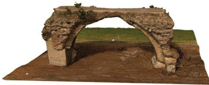
Fig. 3. Perspective view of the arch of the bridge, obtained by the generated point cloud.
