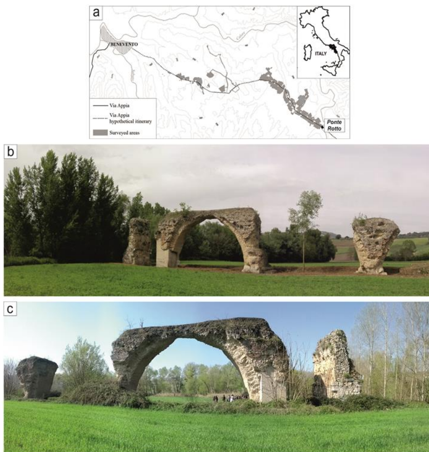
Fig. 1. Sketch map of Ponte Rotto location (modified from [33]); view of western (b) and eastern (c) side of Ponte Rotto.
