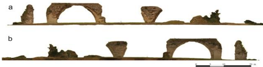
Fig. 5. Lateral orthoimages showing the western (a) e eastern front (b) of Ponte Rotto
