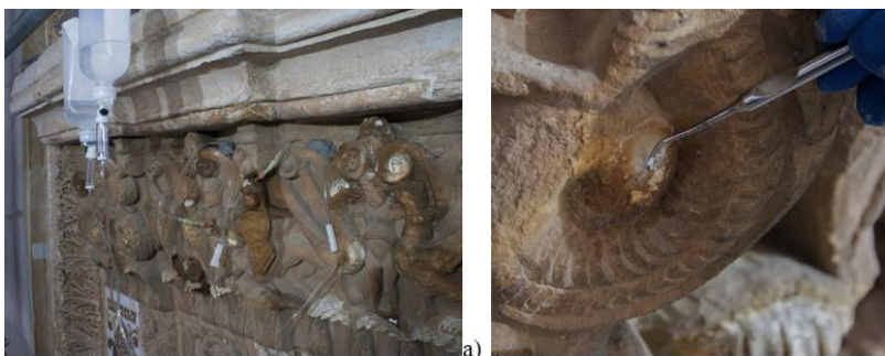
Fig. 9. Particular of capitals. Mineral consolidation treatment with di-ammonium phosphate solution applied by a slow drip. Consolidation treatment of a fissure made by using a lime mortar added with di-ammonium phosphate solution.
