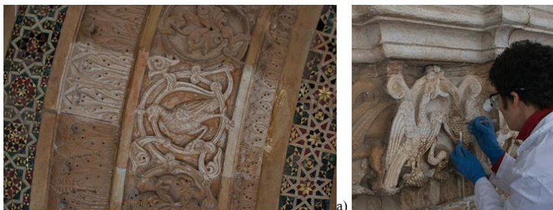
Fig. 8. a) Particular of the archivolt. Cleaning test of polychrome marble surface for removing deposits, black crust and coverings. b) Particular of a capital. Cleaning treatment carried out with surgical scalpel and magnifying eyeglasses.
